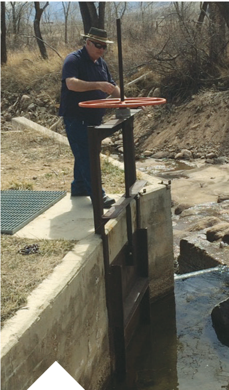
This is one of several improved irrigation diversion structures. Note that the water level is higher, enabling water to easily run through the gate when it is opened. There also are boulders placed in front of the gate to decrease the amount of debris that goes down the ditch.
